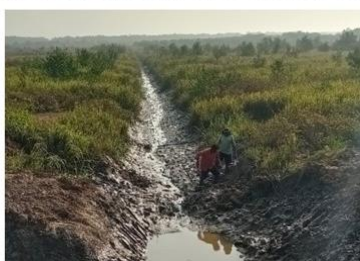
Figure 6: Creek Deepening of 2kms near Bagapatia, Bhitarkanika Landscape
